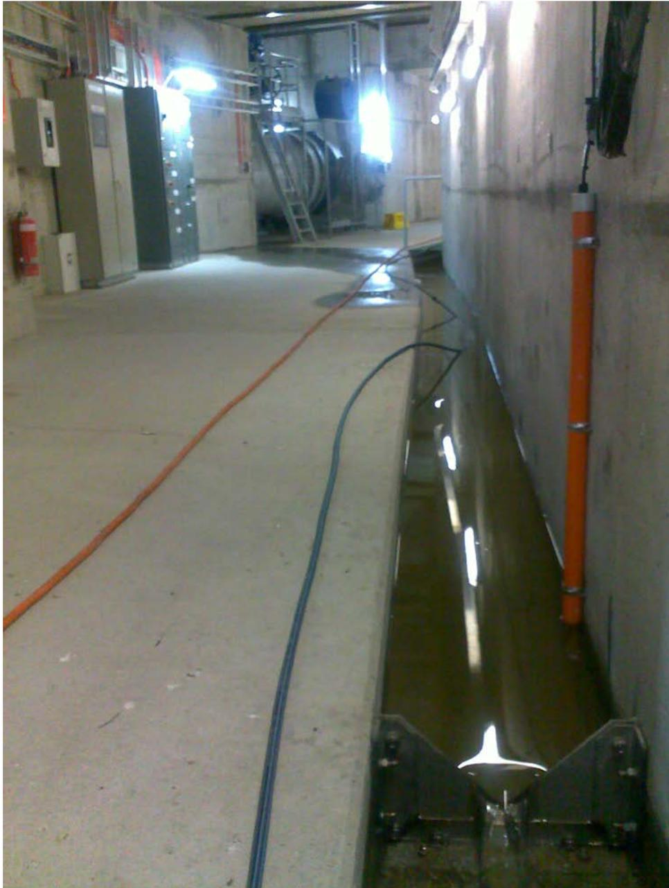
V-notch weir enabling measurement of volume flow leakage from gallery
