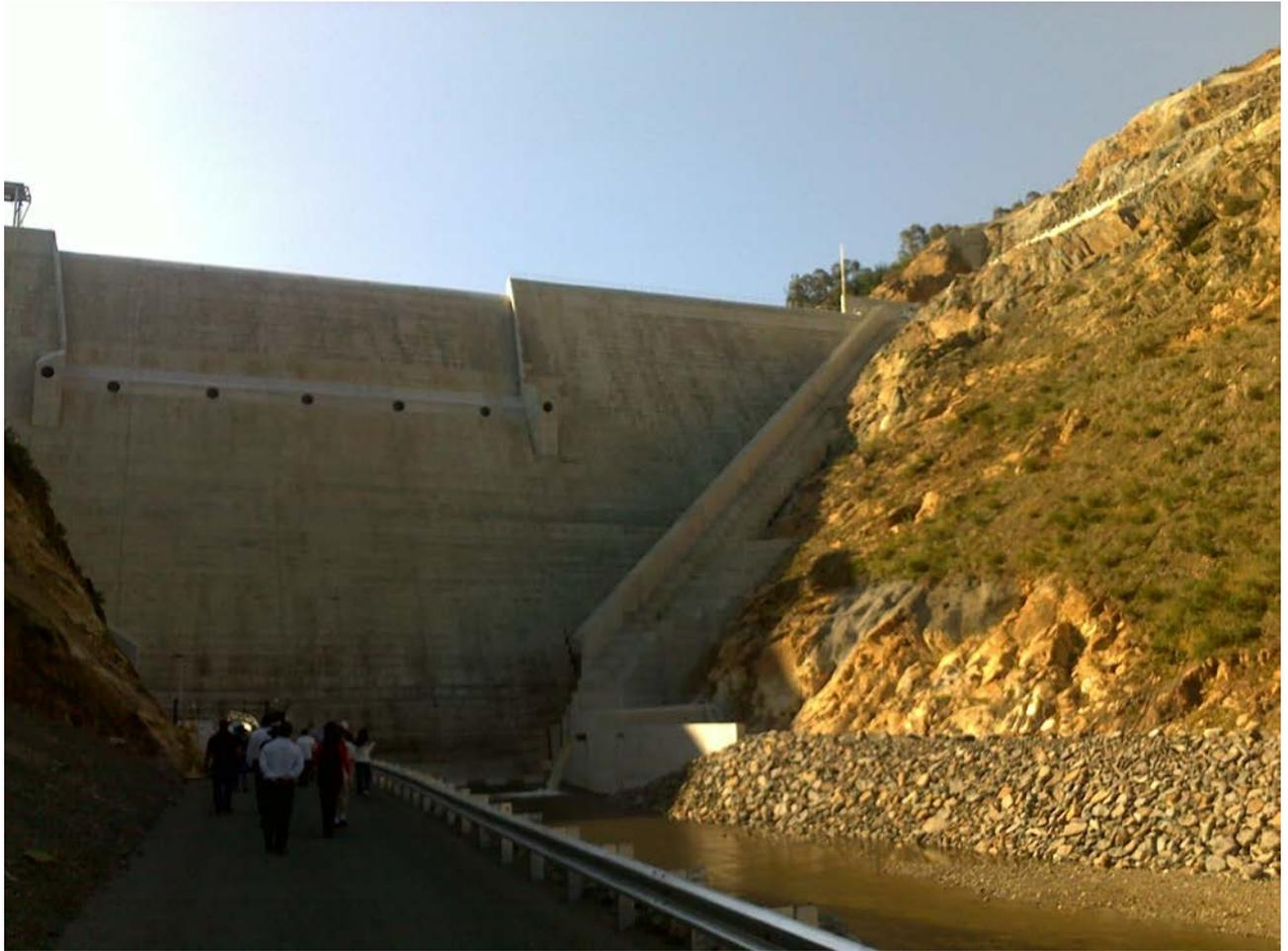
Spillway and dam wall are designed to introduce turbulence during high flows to reduce energy and thus downstream erosion.
