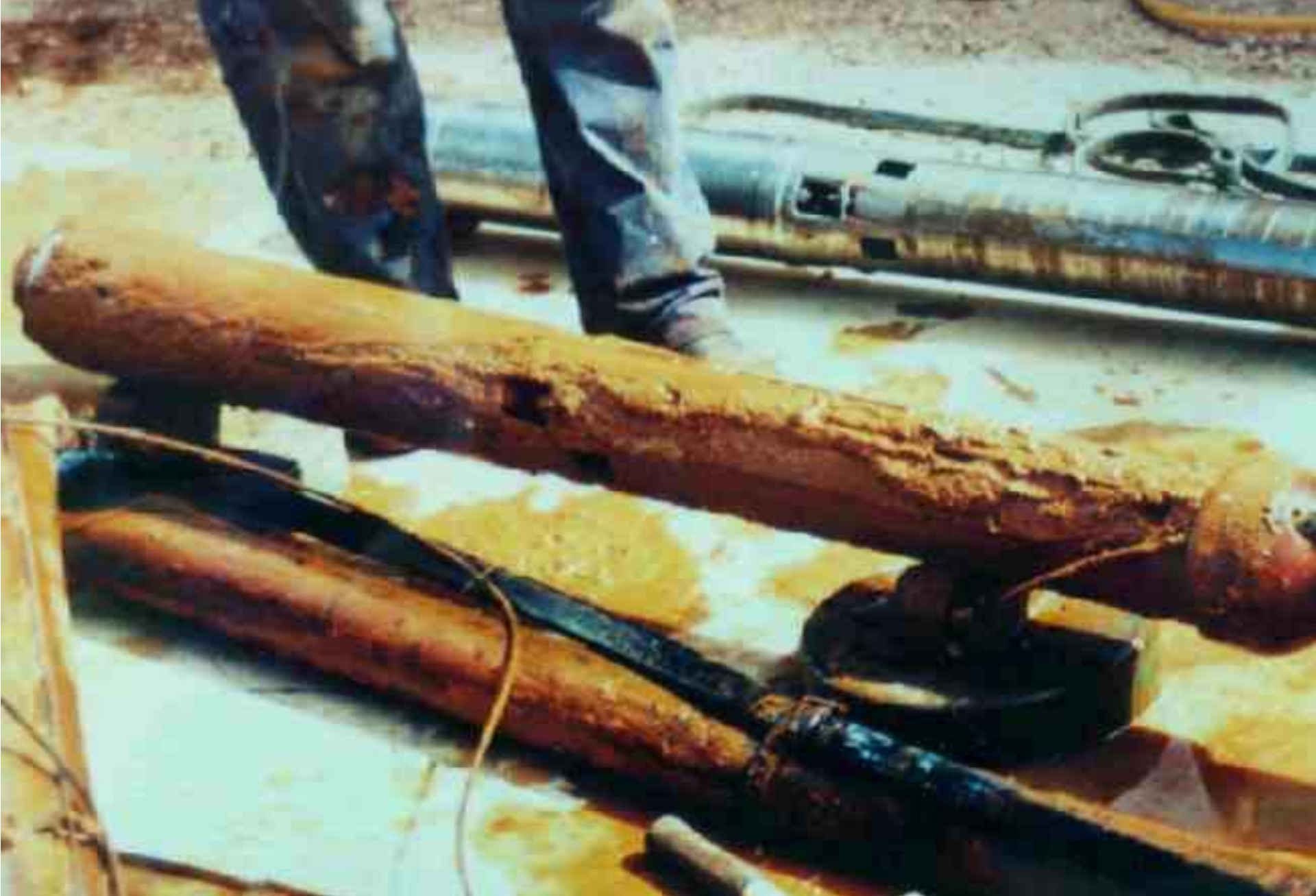
Woolpunda SIS - Iron Bacteria Covered Pump Being Removed
