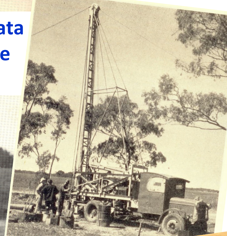
Fig. 17.—The Percussive "Dimboola No. 1" Borehole
