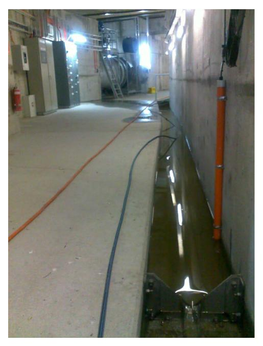
V-notch weir enabling measurement of volume flow leakage from gallery
