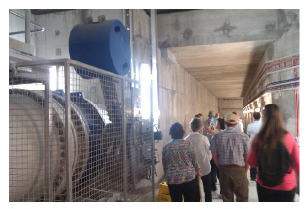
Dam outlet shut off valve with levered counterweight to prevent water hammer
