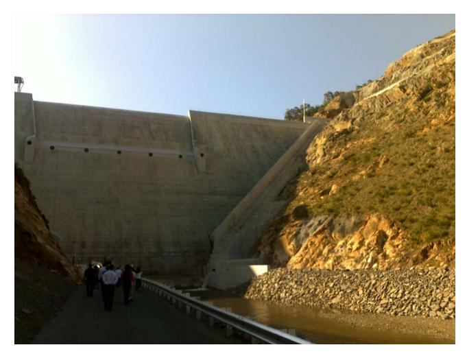
Spillway and dam wall are designed to introduce turbulence during high flows to reduce energy and thus downstream erosion.
