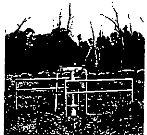
A rehabilitated artesian bore showing valves to control flow, pipes to reticulate water and a fence for protection from stock.
